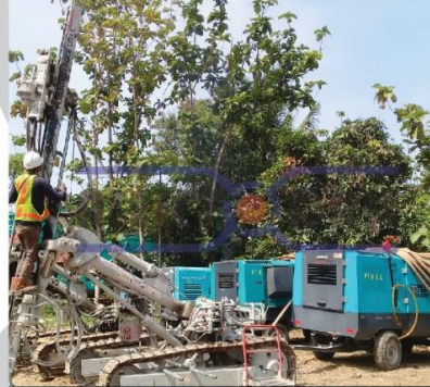
Drilling Blasting Purwakarta, Jawa Barat
