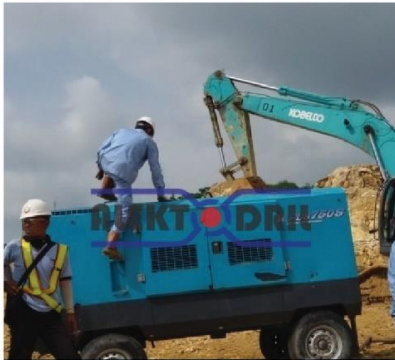
Drilling Blasting Pekerjaan Quarry, Bayah
